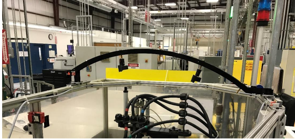
Figure 11. Microphone bracket (SD506017) secured in position over test station
