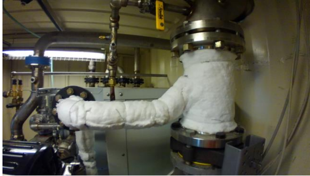
Figure 5 Thermal barrier installed
