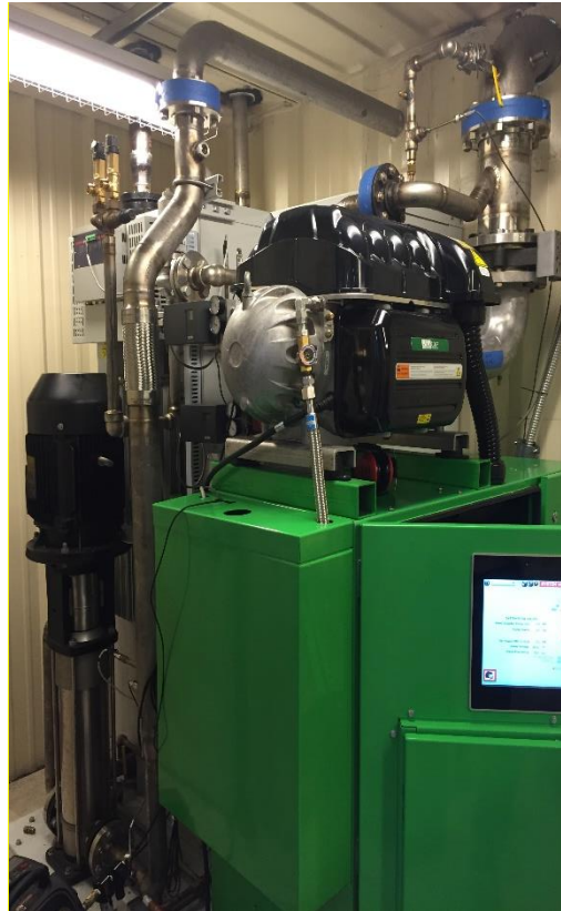
Figure 19. View of the ORC Components
