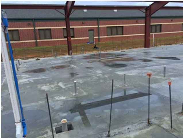
Figure 22: Example Construction Site
