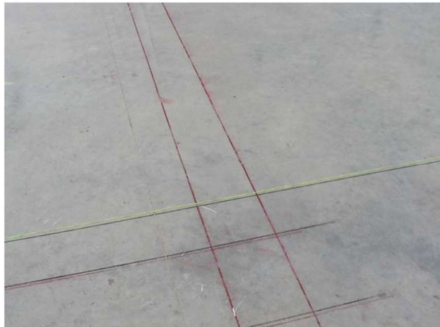
Figure 11 – Example Construction Marks
