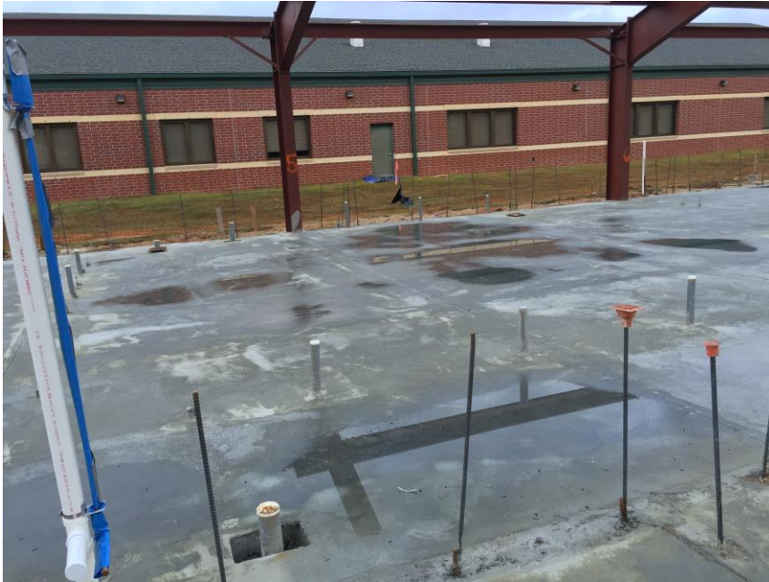
Typical construction site
