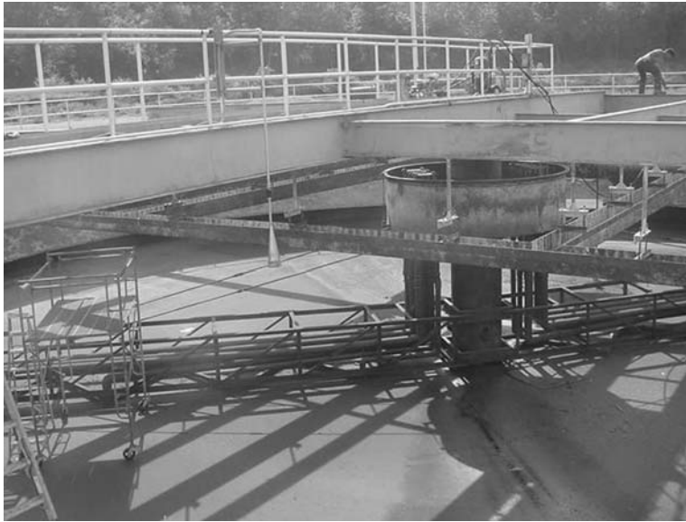
FIGURE 10.5 Ultrasonic sludge blanket level detector (published with permission of Siemens-Milltronics, New York).
