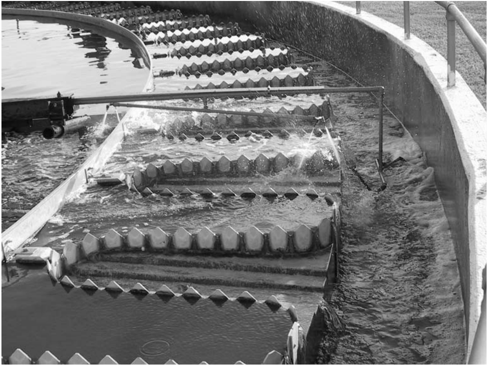
FIGURE 8.43 Water spray jet system removing algae from serpentine weirs.
