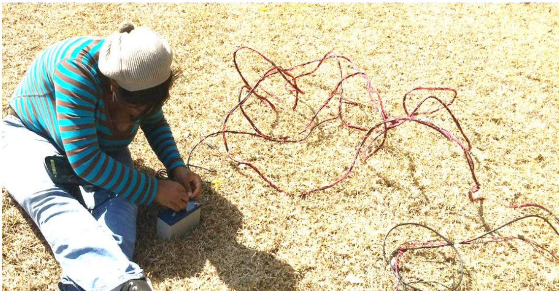
Figure 17 Preliminary testing of the electrical components
