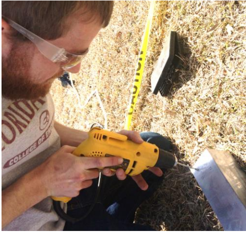
Figure 20 Thomas drilling holes in the poles to fit the brackets
