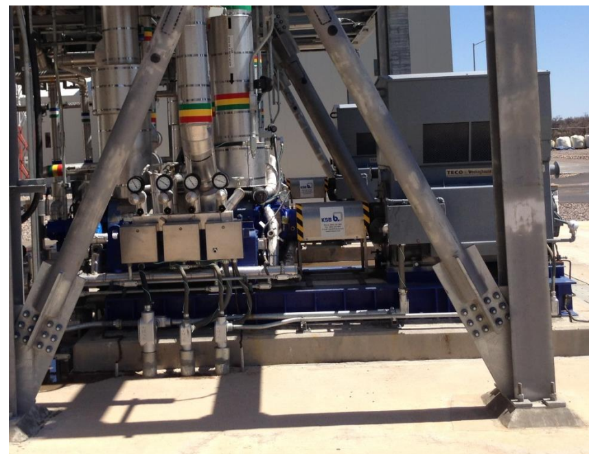
Typical BFP – Monitor for abnormal temps
