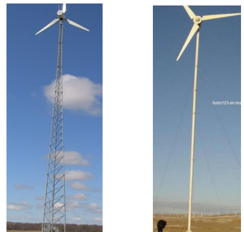
Figure 4.2.2 Photographs of lattice tower (left) and steel tubular tower
