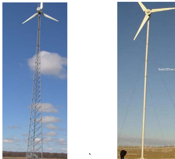
Figure 3.2.2 Photographs of lattice tower (left) and steel tubular tower (right)
