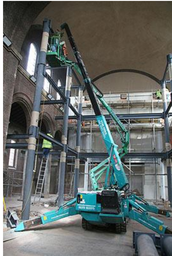
Figure 2 – Retractable support struts on a crane performing construction in a church.
