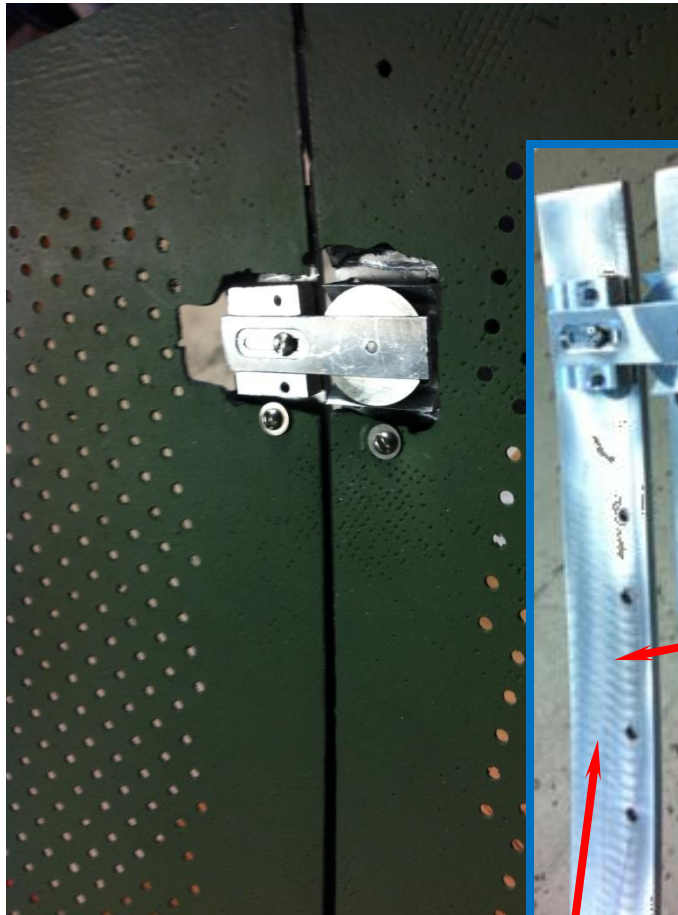
Panel-to-Panel interlocking
