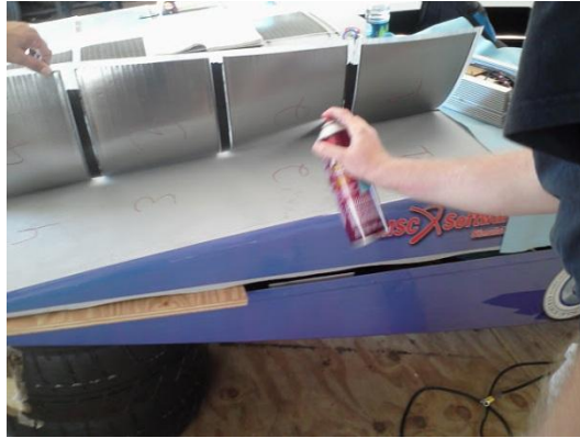
Figure 24 - Mounting modules with spray adhesive and mounting tape (color-coded placement).
